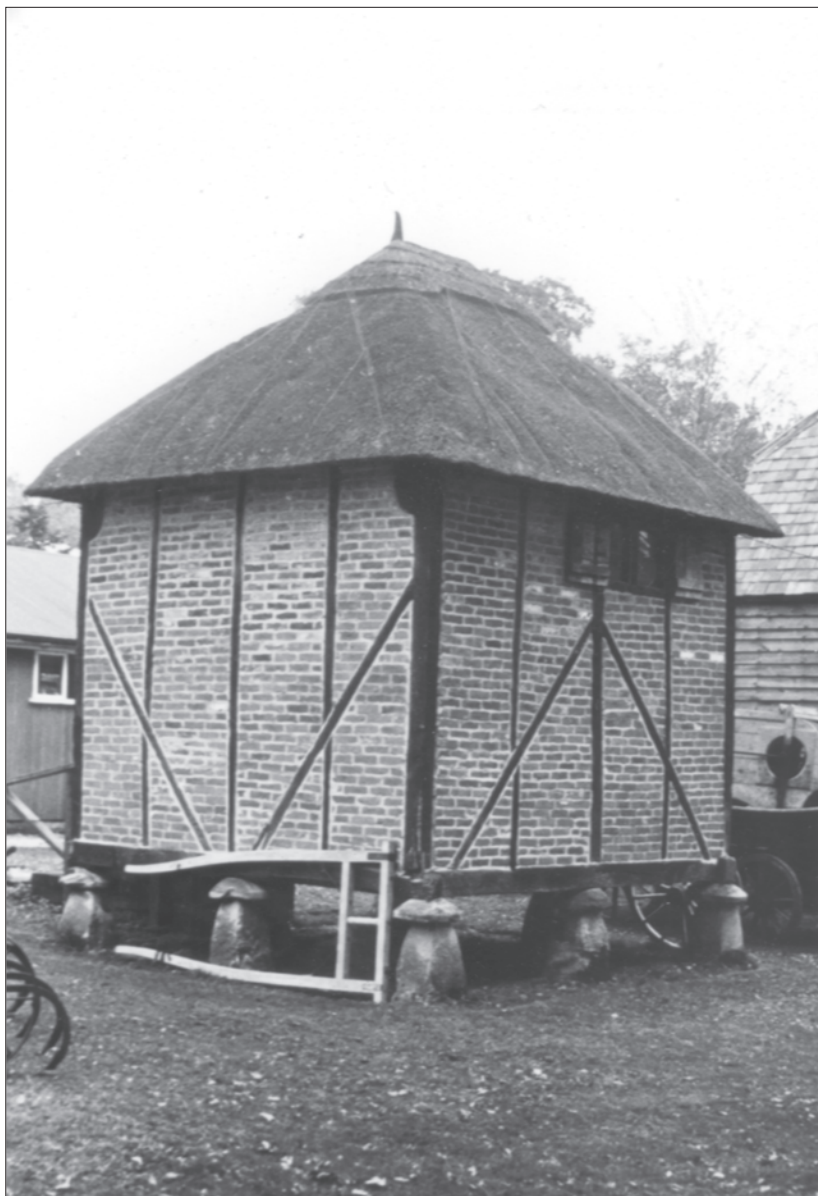
A granary raised on staddle stones to prevent rats and mice gaining entry. This was formerly in the Longleat estate, and has been moved to Lackham Museum of Agriculture and Rural Life, Wiltshire College Lackham.
