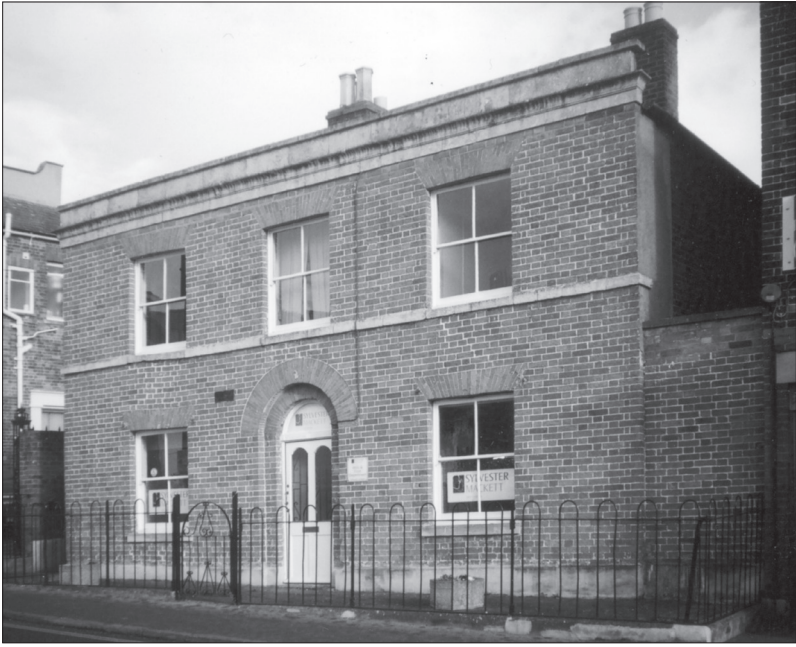
No. 61 Castle Street, where Tucker was brought up
