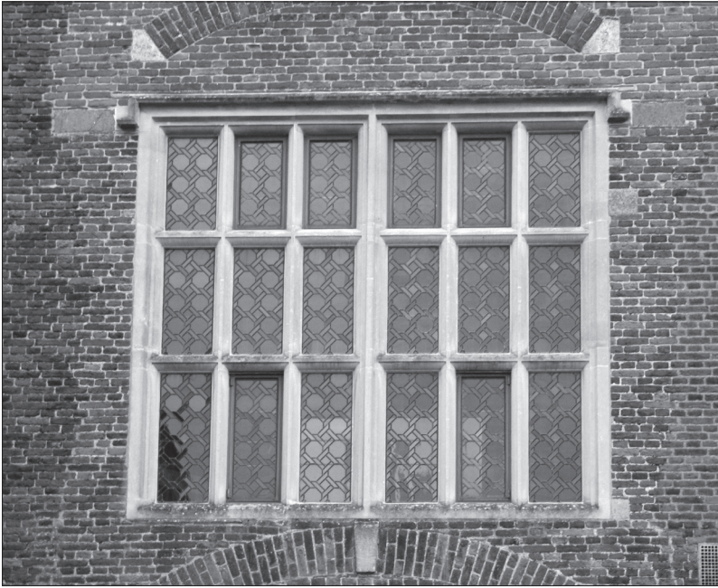
Window (opposite page) at seventeenth-century Joiners' Hall, illustrated in Peter Hall's Picturesque Memorials, copied by William Small for new window (above) at the rear of The King's House, now Salisbury & South Wiltshire Museum. Photo Joe Newman
